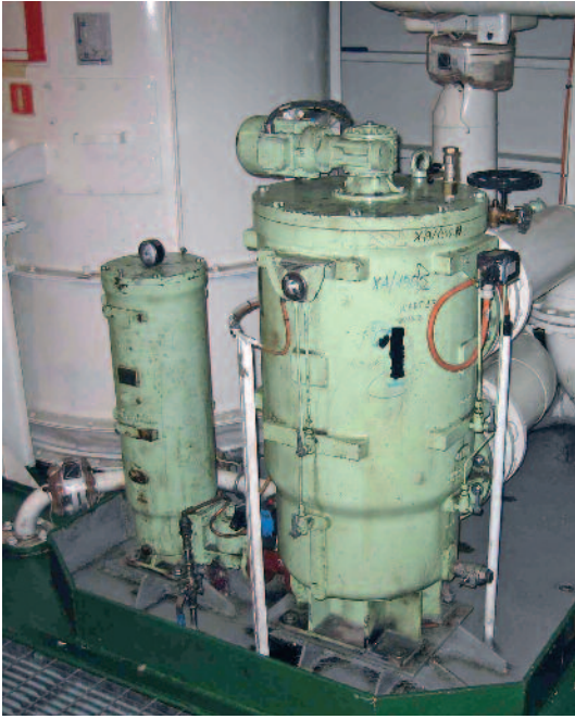
4-Stroke Diesel Marine Engine WÄRTSILÄ 12V46 Ship "MOBY AKI" ACX-RM Filter - Filtration 35 µm
