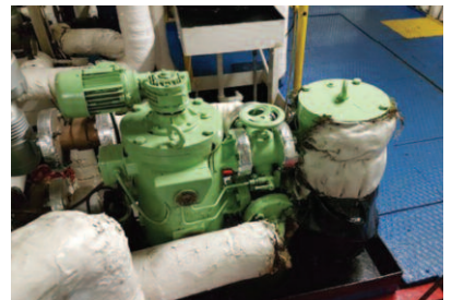
Booster System Diesel Engine PIELSTICK 12PC3V480 Ship "M/T DREA" DACT Filter - Filtration 25 µm absolute
